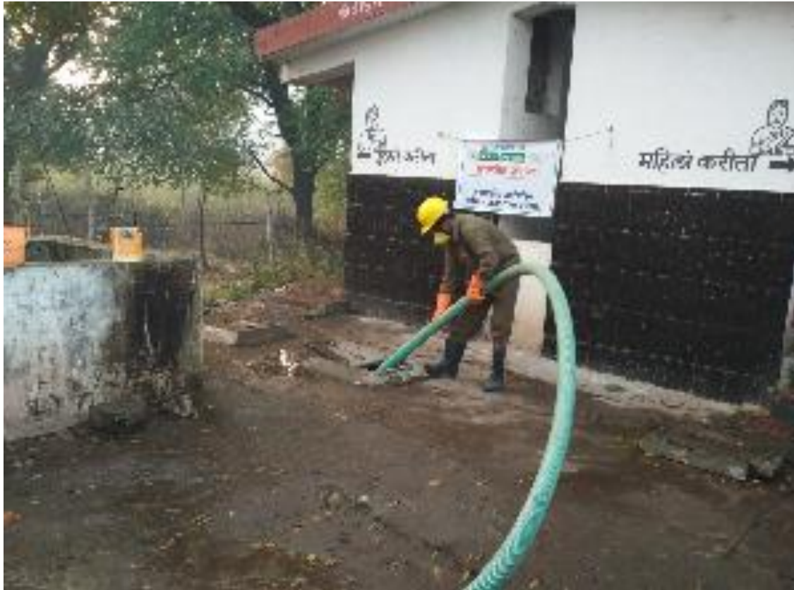
Step 1: Install hose in septic tank
