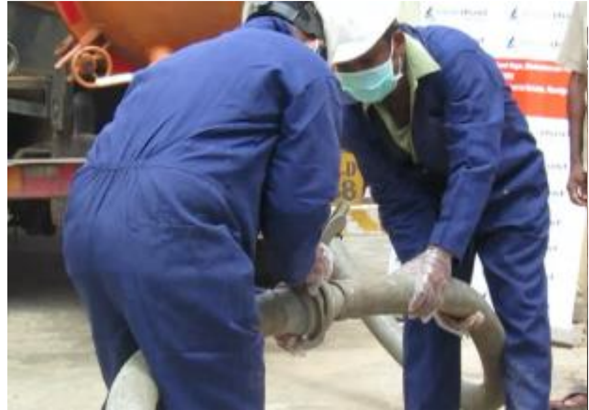
Step 4: Connect hose pipe to the truck
