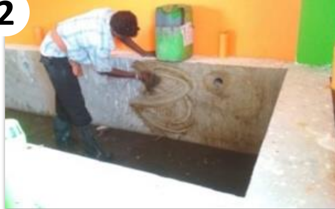
Preparing composting pits
