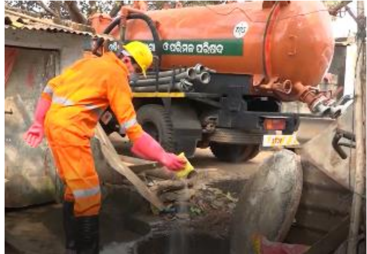
Step 2: Add chlorine in the septic tank
