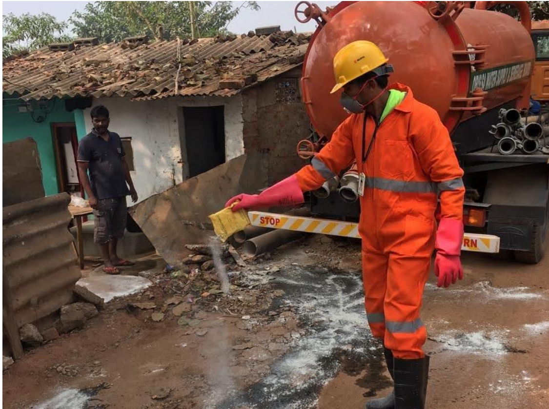
Step 7: Add lime on hose after emptying
