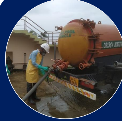
Workers in Operation and Maintenance of Deep Row Entrenchments / Fecal Sludge Treatment Plants
