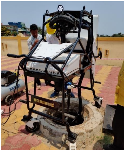
Video (01:48): https://bit.ly/3yKqfCs Use of sewer cleaning robot
