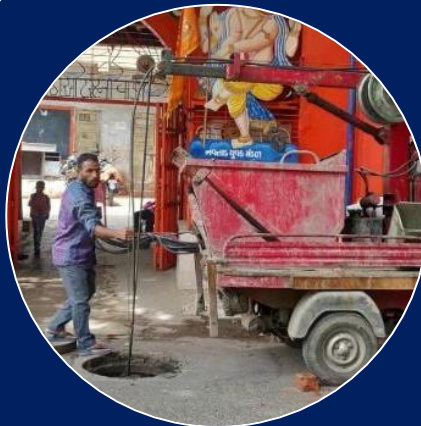
Maintenance hole /sewer lines cleaners
