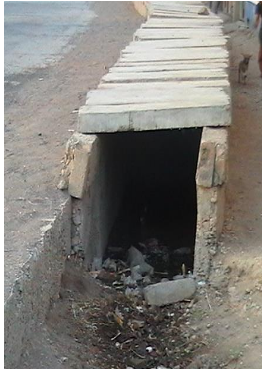
Covered (Box) Drain
