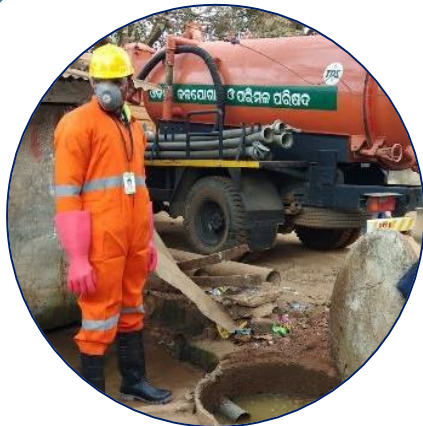
Desludgers - emptying of septic tanks/pits
